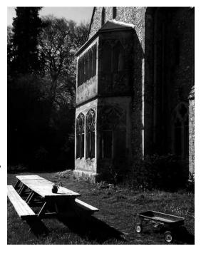
And the wooden buttresses that propped up the double-bay window for over 25 years have now been removed, because the bay is now reinforced with a stainless steel "trouser belt'' - at a cost of only £1,300 instead of the threatened £75,000. The house is returned to its former glory at last.
